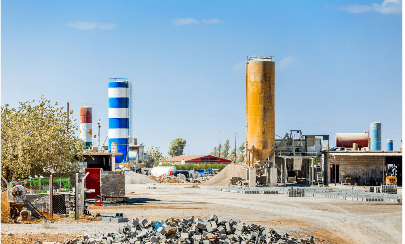
Old concrete batch plant in Erbil, Iraq. August 13, 2016. Shutterstock
